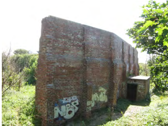
(left), Rifle Range, (WW2 (Kings L.pool Regiment), The King's main depot was here in Formby at Harington Barracks throughout the second World War. Rifle practice took place on this open range , later at Altcar Rifle Range, This is our only surviving structural reminder of the King's Liverpool Regiment.
