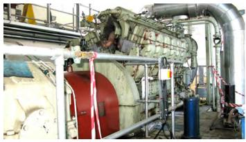
The pump that failed -the drive to the impellor is in the foreground.; photo Jack
